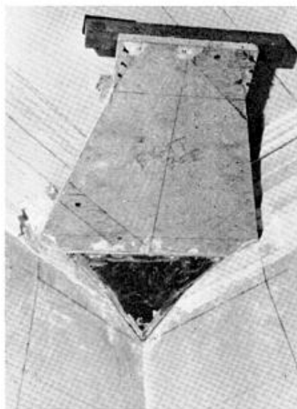
Fig. 4 (above) shows upper part of throat section fixed to corner and ceiling.
