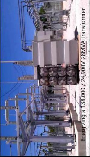
Energizing a 138,000 / 24,900V 28MVA transformer
