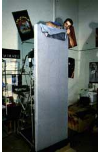
The grill cloth is stretched over the frame and stapled at top and bottom.
